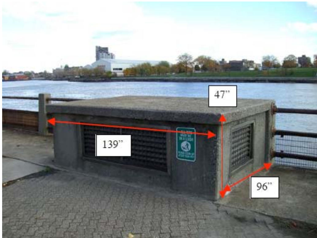
Photo 4.3.8.2-1. Typical existing steam tunnel vent.
