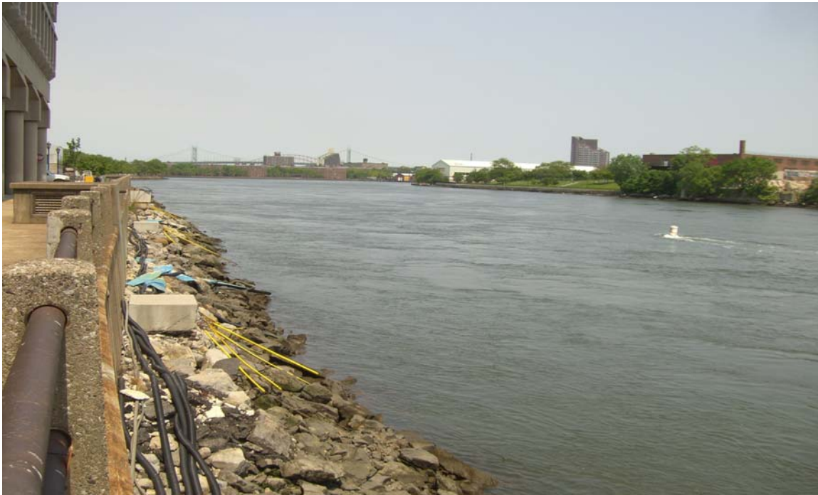
Photo 4.3.6.1-2. From RITE Control Room, looking toward Hallet's Cove
