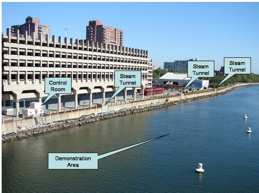
Photo 4.3.8.1-1. Verdant Power RITE Demonstration Site, buoy system, control room, and nearby steam tunnel vaults.
